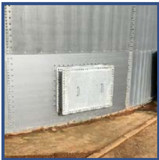
Rectangular access hatch 920 mm x 600 mm
